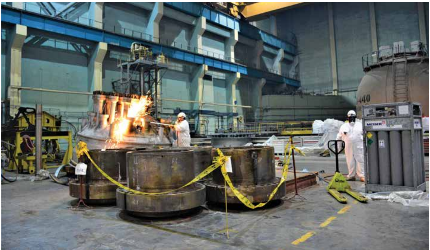
Size reduction of an upper block cap by means of oxy-fuel cutting, Photo SE RAW
