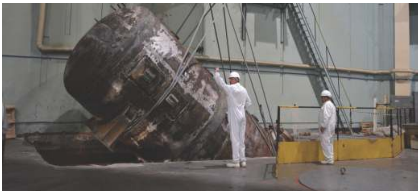
Dismantling of steam generator of Unit 3, Photo SE RAW
